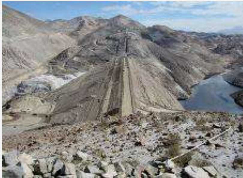
TSF Initial Starter Dam Construction
