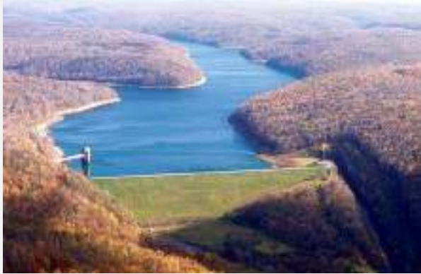
East Branch Dam; Elk Co., PA
