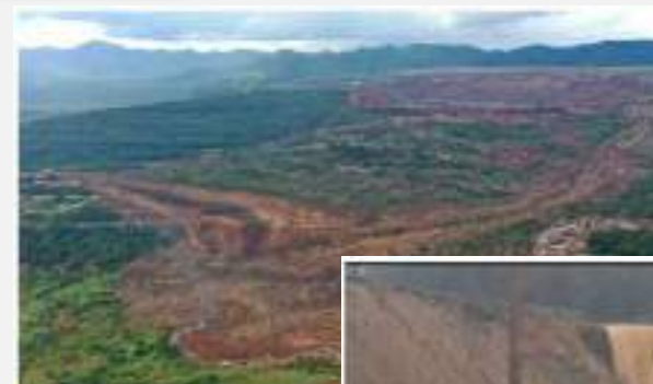
The 4 November 2025 Landslide at Mae Moh Mine in Thailand
